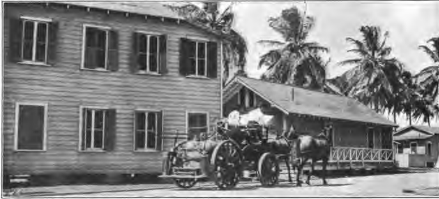
Chemical Engine, part of the Equipment of the American Fire Department of the Canal Zone.
