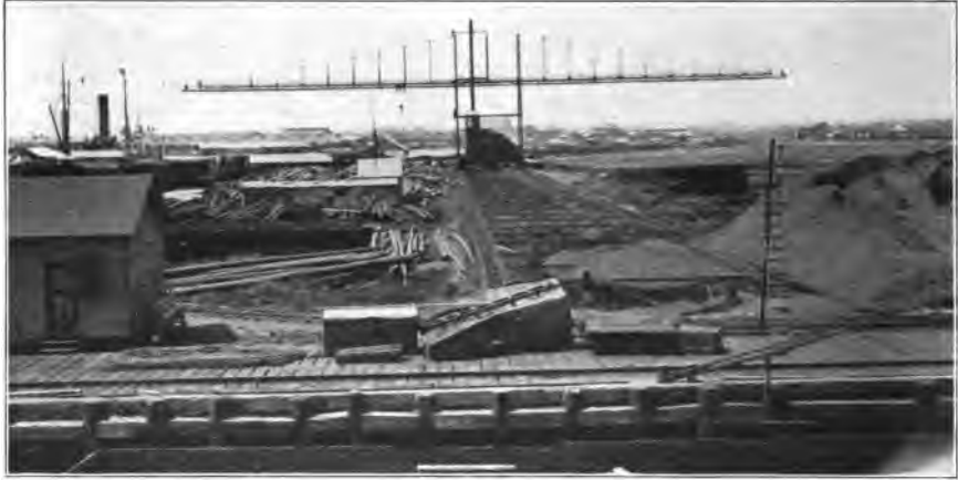
An Unloading Crane or Hoist used in the work of the Canal.
